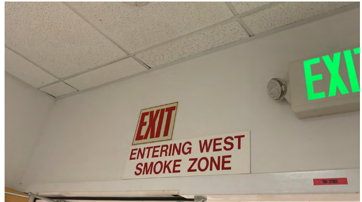
Signage indicating smoke zones, which are separated by a smoke barrier.
