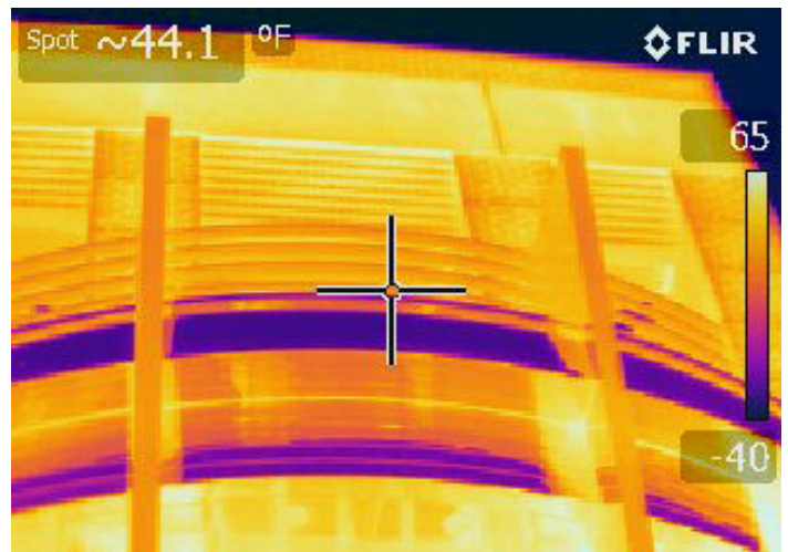
Building enclosure thermal imaging.
