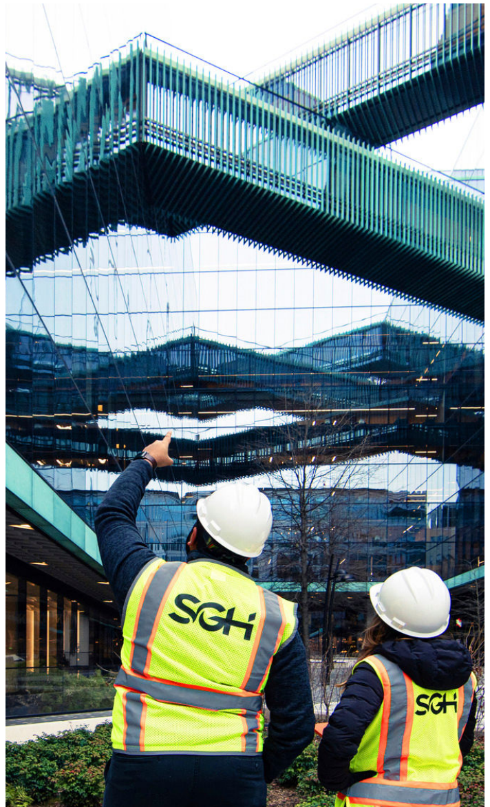
Construction site observations.
