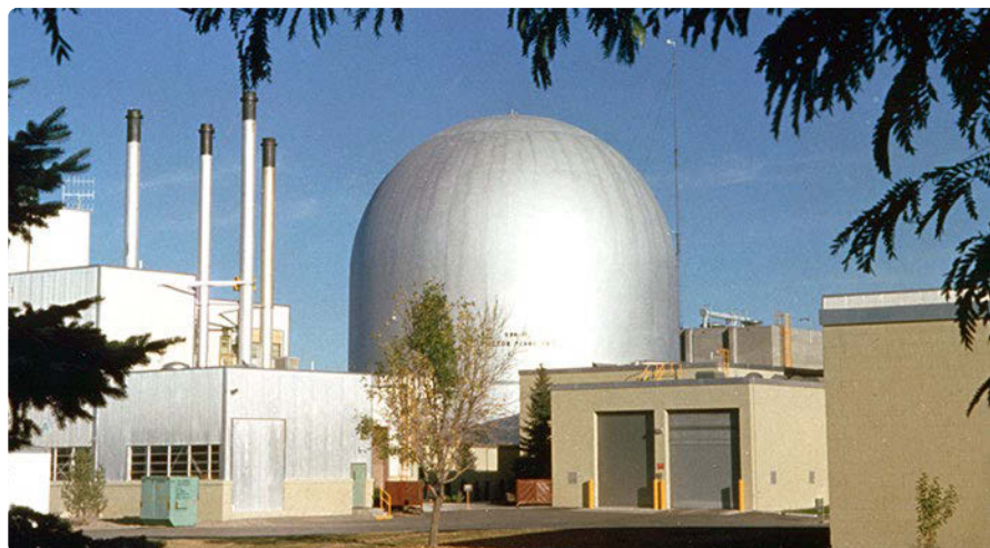
The National Reactor Innovation Center's Demonstration of Microreactor Experiments (NRIC DOME) microreactor test bed at INL. (Photo: DOE)
