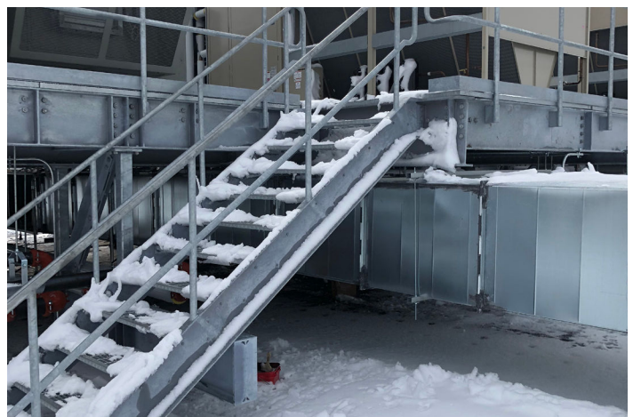
The code now considers snow accumulating on open-framed structures, such as grating.
