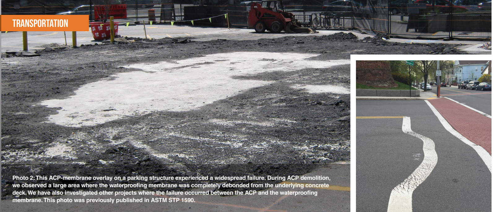
Photo 1: This roadway ACP failed a few months after placement. The top ACP top course was not well bonded to the ACP binder course below. The top layer moved laterally 2 feet due to shear stresses from vehicle braking forces.
