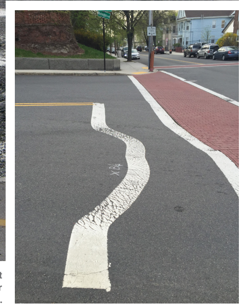
Photo 1: This roadway ACP failed a few months after placement. The top ACP top course was not well bonded to the ACP binder course below. The top layer moved laterally 2 feet due to shear stresses from vehicle braking forces.
